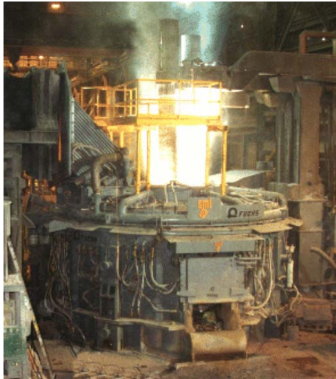
Fig. 2.2 Operating Electric Arc Furnace
