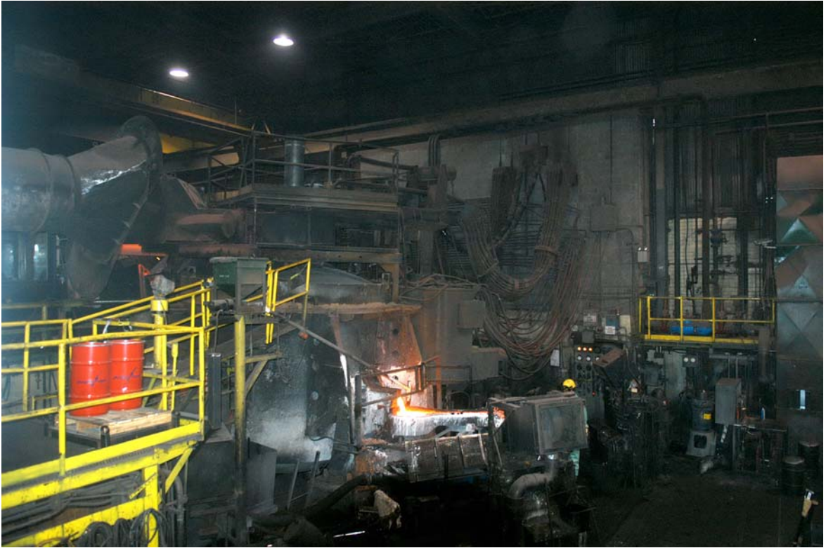
Fig. 2.3 Subject Electric Arc Furnace in operation
