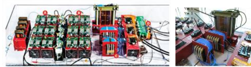
(b) Pictures with AC-link transformers (2009)
